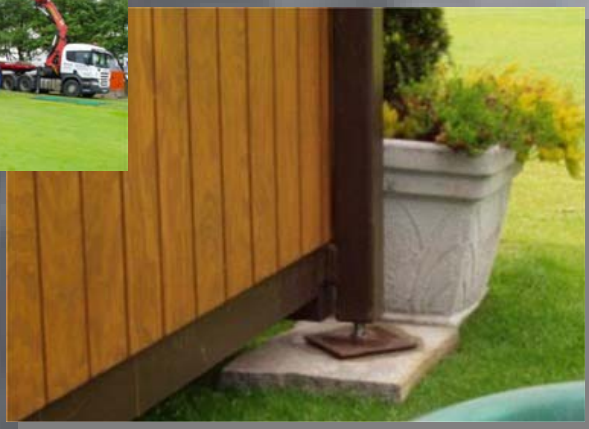
Easily installed on any surface, the legs are adjustable and the feet rest on a small slab providing adequate ground clearance to protect any grass, ventilation and offering an easy and safe route for cabling.
